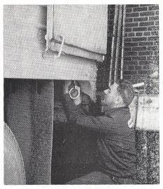
SECURING CONNECTION—Ottomar Rupprecht, Bottling Maintenance Department, fastens bolts to transport truck in making safe-loading connection with our newly-developed safety chock and security chain.
