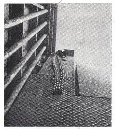
SO IT WON'T BUDGE—This photo shows a husky log chain, 15 feet long and of three-eighths-inch steel links used on the loading dock of our plant to prevent trucks from slipping while being loaded.
